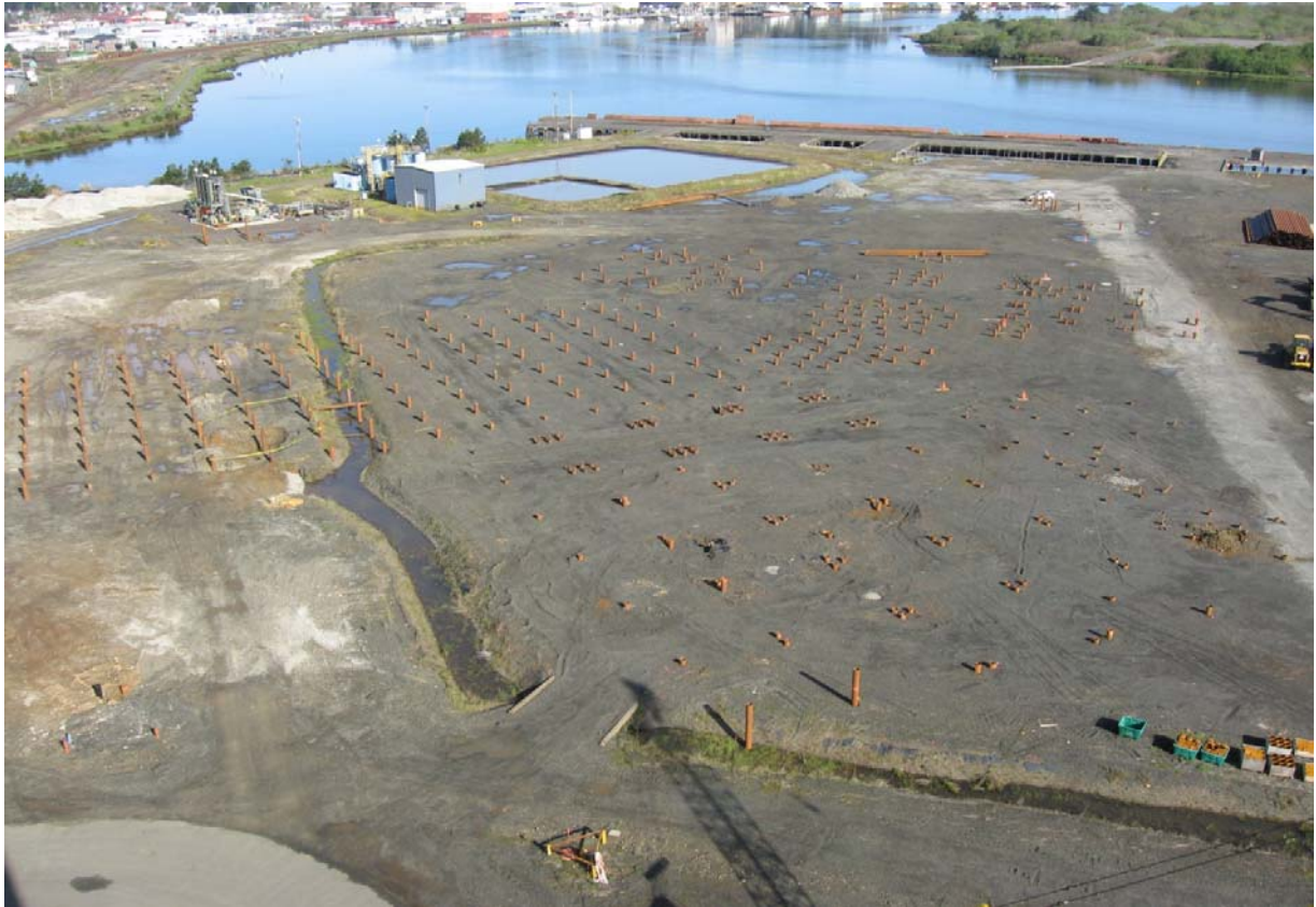
Figure 1: Partial view of processing site depicting completed foundation support pilings
