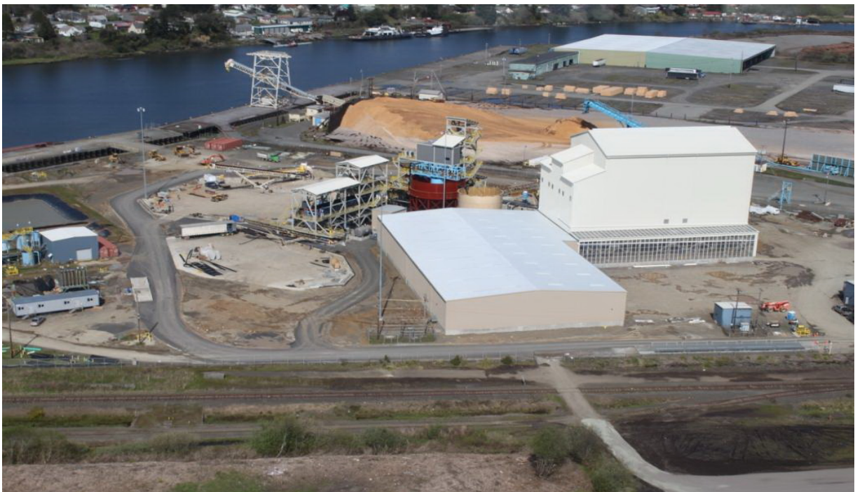
Coos Bay mineral process site 5 April 2011 -- The large covered building in the foreground is the warehouse, the taller structure at 1 o'clock is the dry plant and the wet plant is the open structure at 11 o'clock. The red tank immediately behind the warehouse is the thickener. The water processing and storage facility is at the left of the picture.
